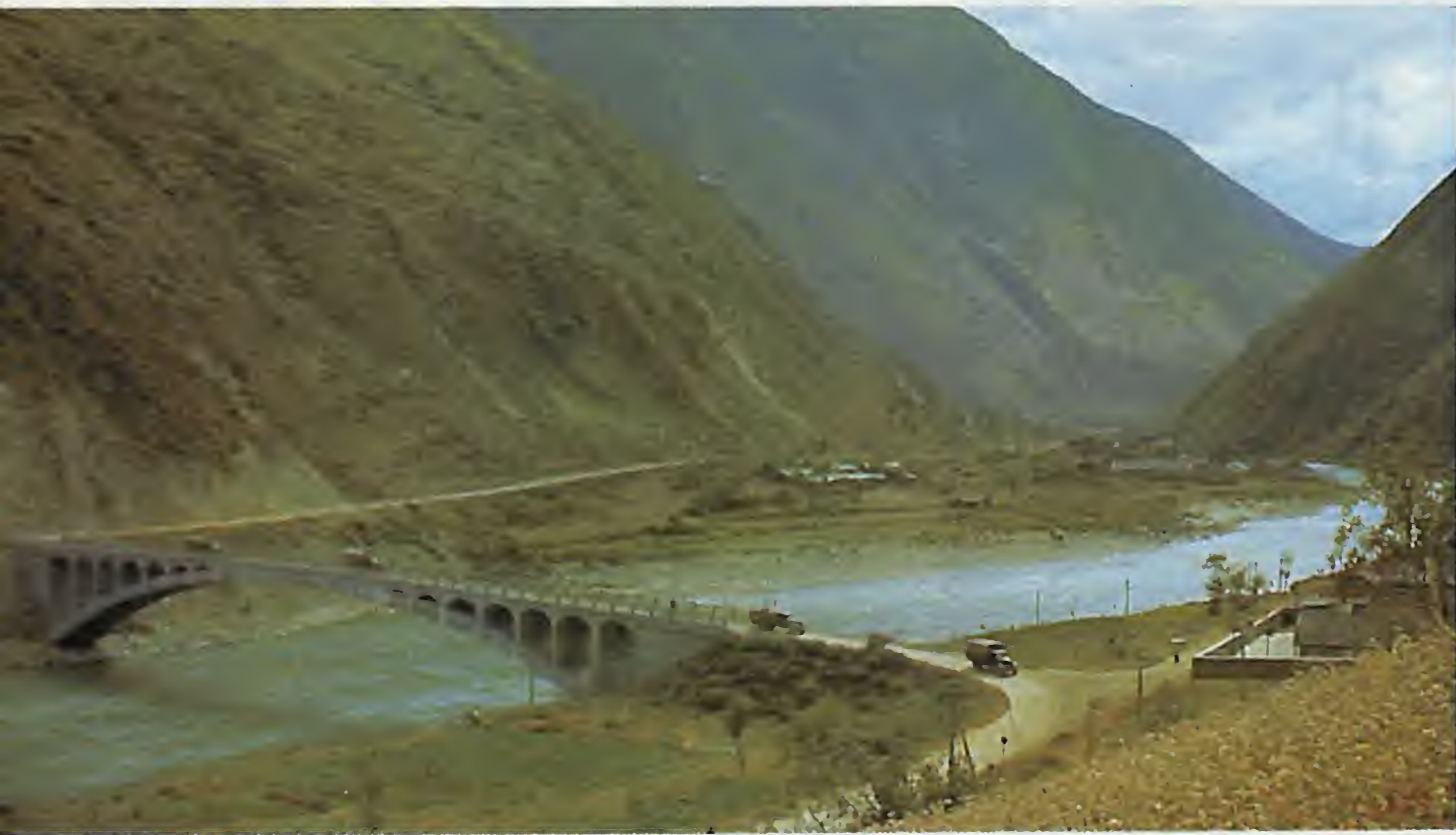
The new Luting Bridge.
